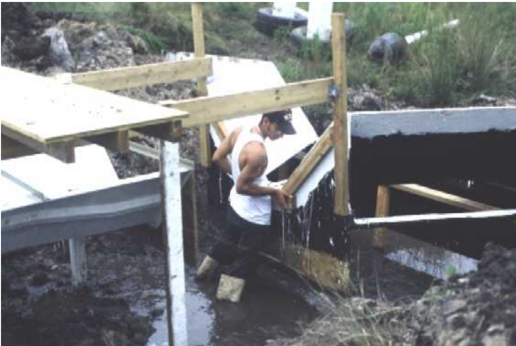
Figure 3.5. Construction of flume station.
