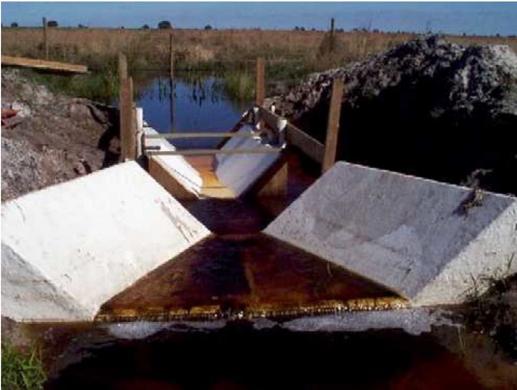
Figure 3.4. Construction of flume station.
