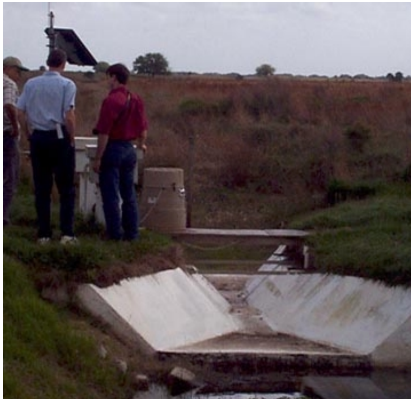
Figure 3.7. Completed flume station.
