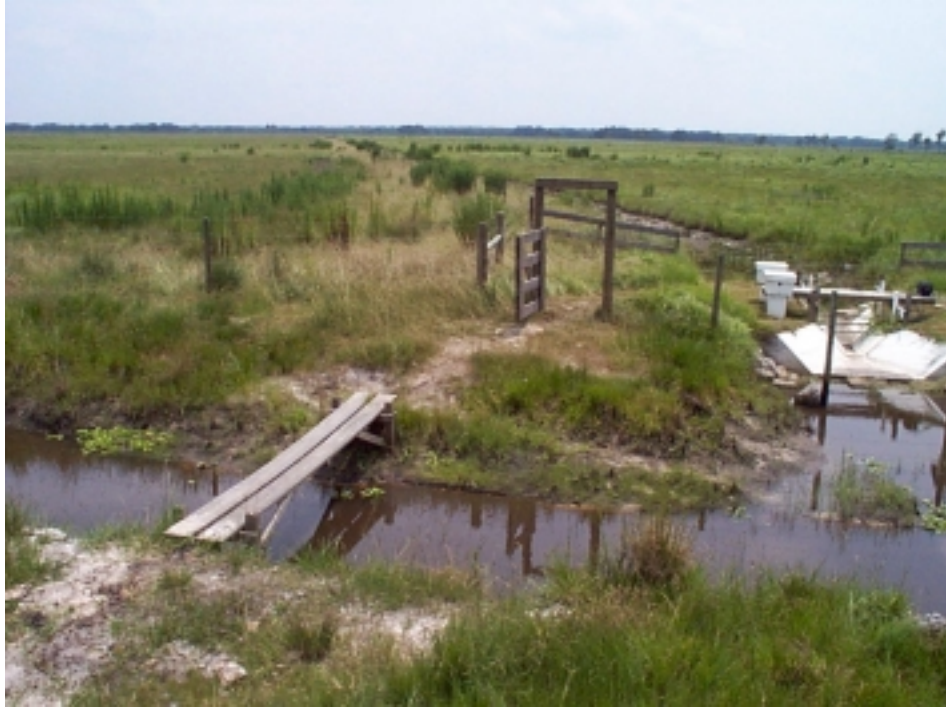
Figure 3.6. View of flume station from downstream location.
